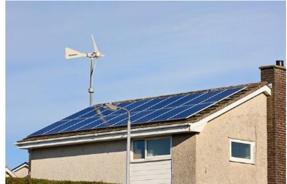
Figure 6. Example of a hybrid wind-photovoltaic system
